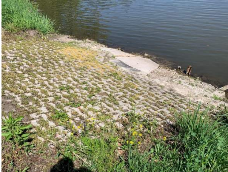
Figure 2.5 Category B – Existing Boat Launch, 4-N
