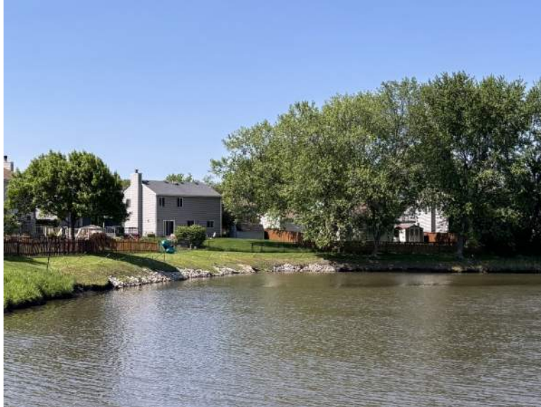
Figure 2.13 Category C – Existing Riprap, 8-S
