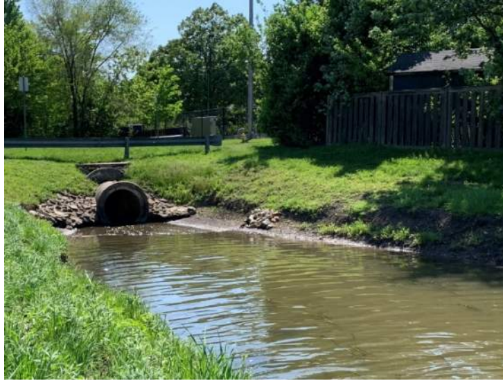
Figure 2.7 Category C – Outlet Culvert, 6-S
