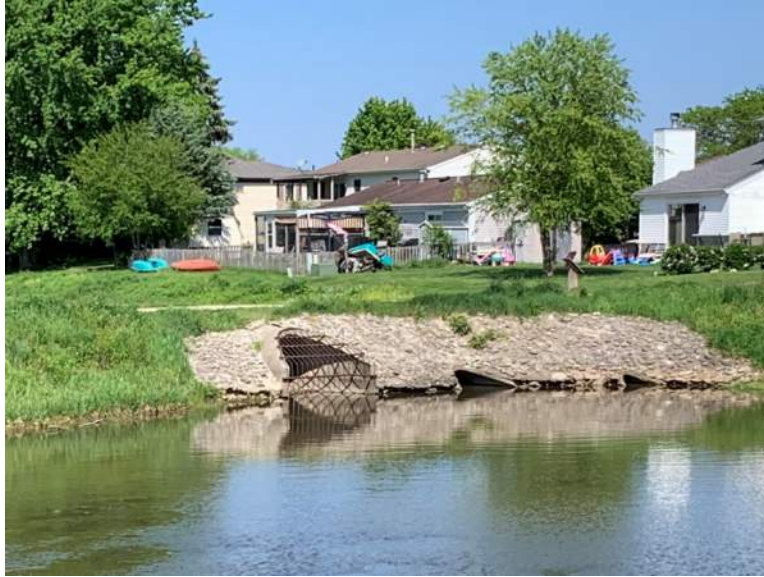
Figure 2.1 Category A – Culverts Between North and South Lakes, 1-5
