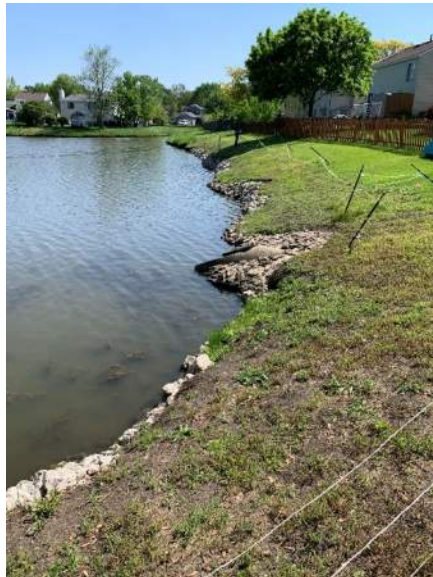
Figure 2.12 Category C – Existing Riprap, 8-S
